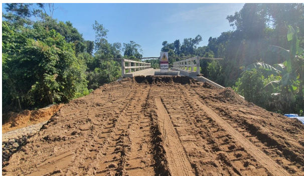
CONST. PUENTE VEHICULAR SIND. VILLA SAN JAVIER D6 VILLA TUNARI
